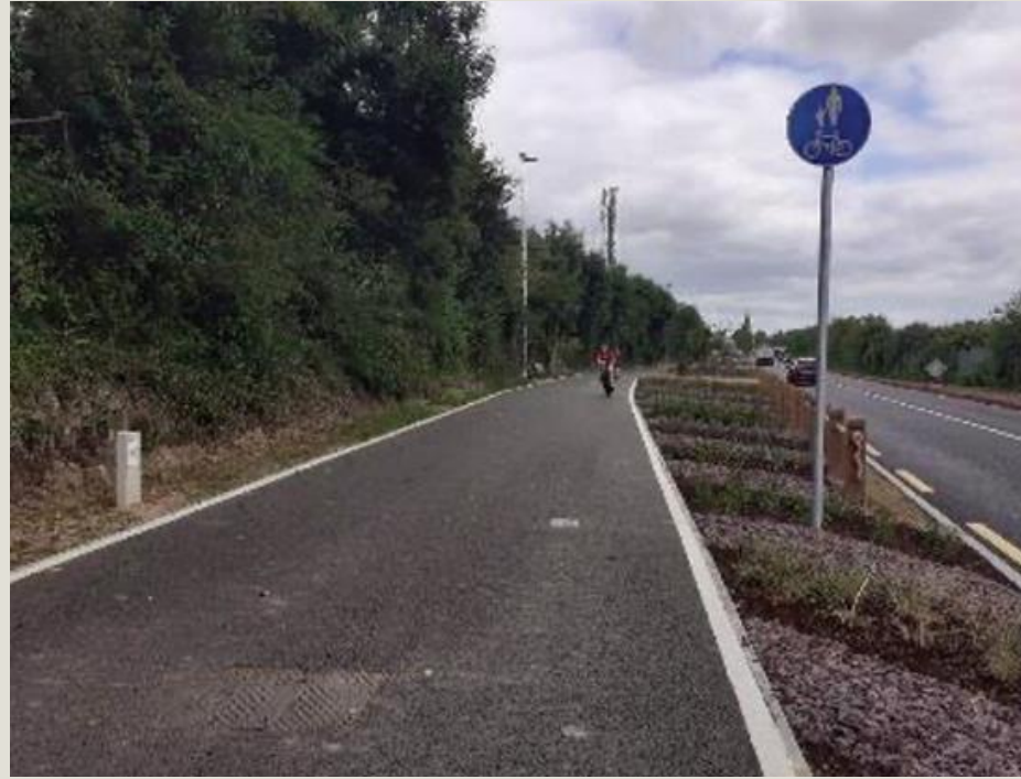
Example of Shared Surface adjacent Carriageway (similar to R132)
